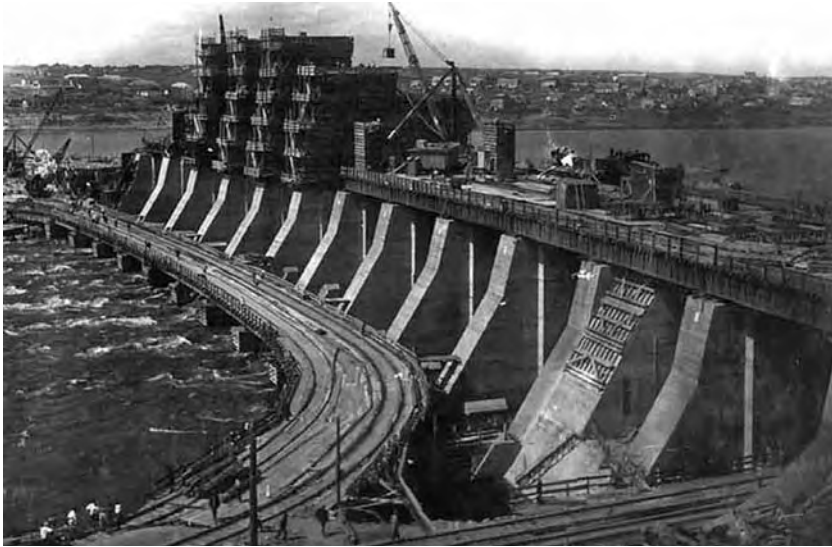
The First Five-Year Plan: A hydroelectric dam in construction
